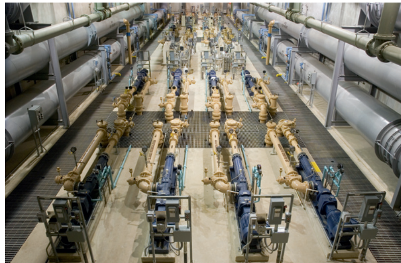
55 seepex range BN 130-6L pumps installed for handling sludge created in the DensaDeg units in Toledo.
